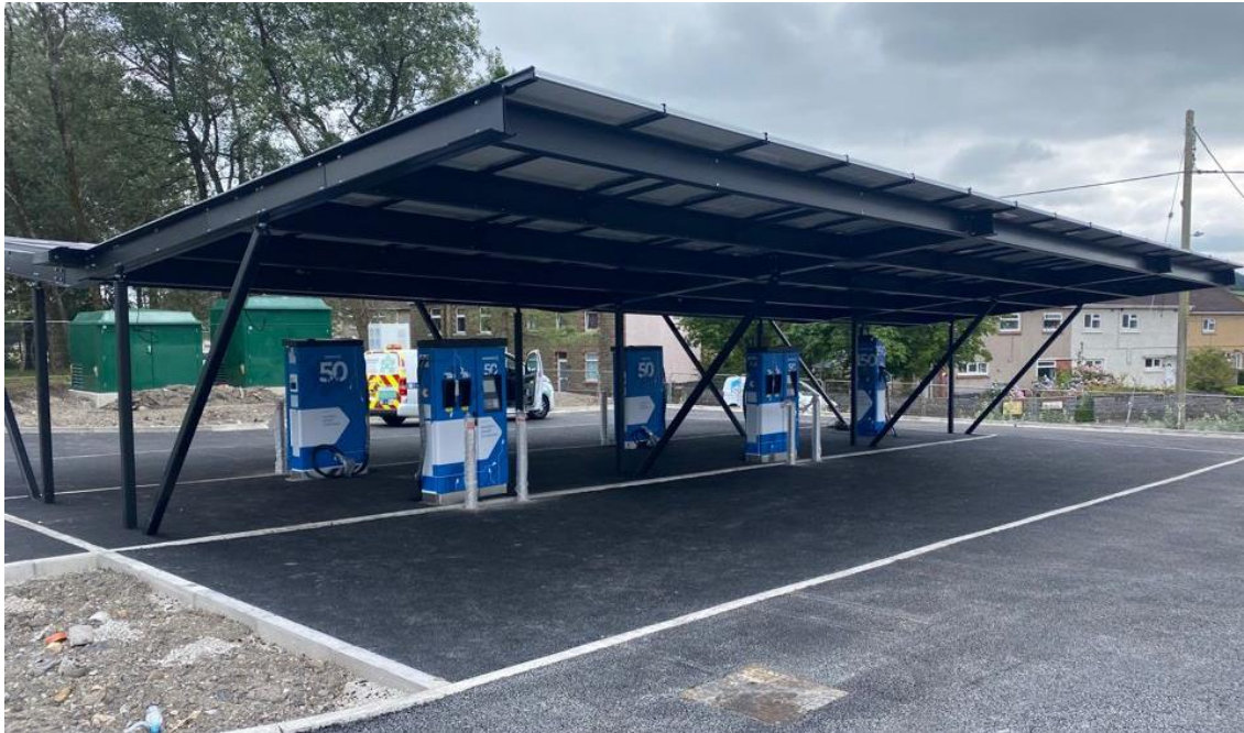
Figure 16 - Cross Hands EV Charging Hub (in construction)
